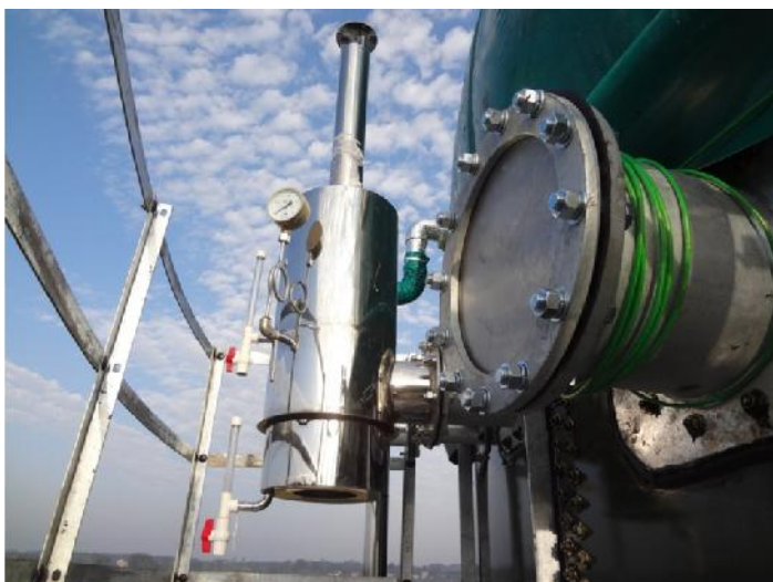
Over/under pressure protection device
